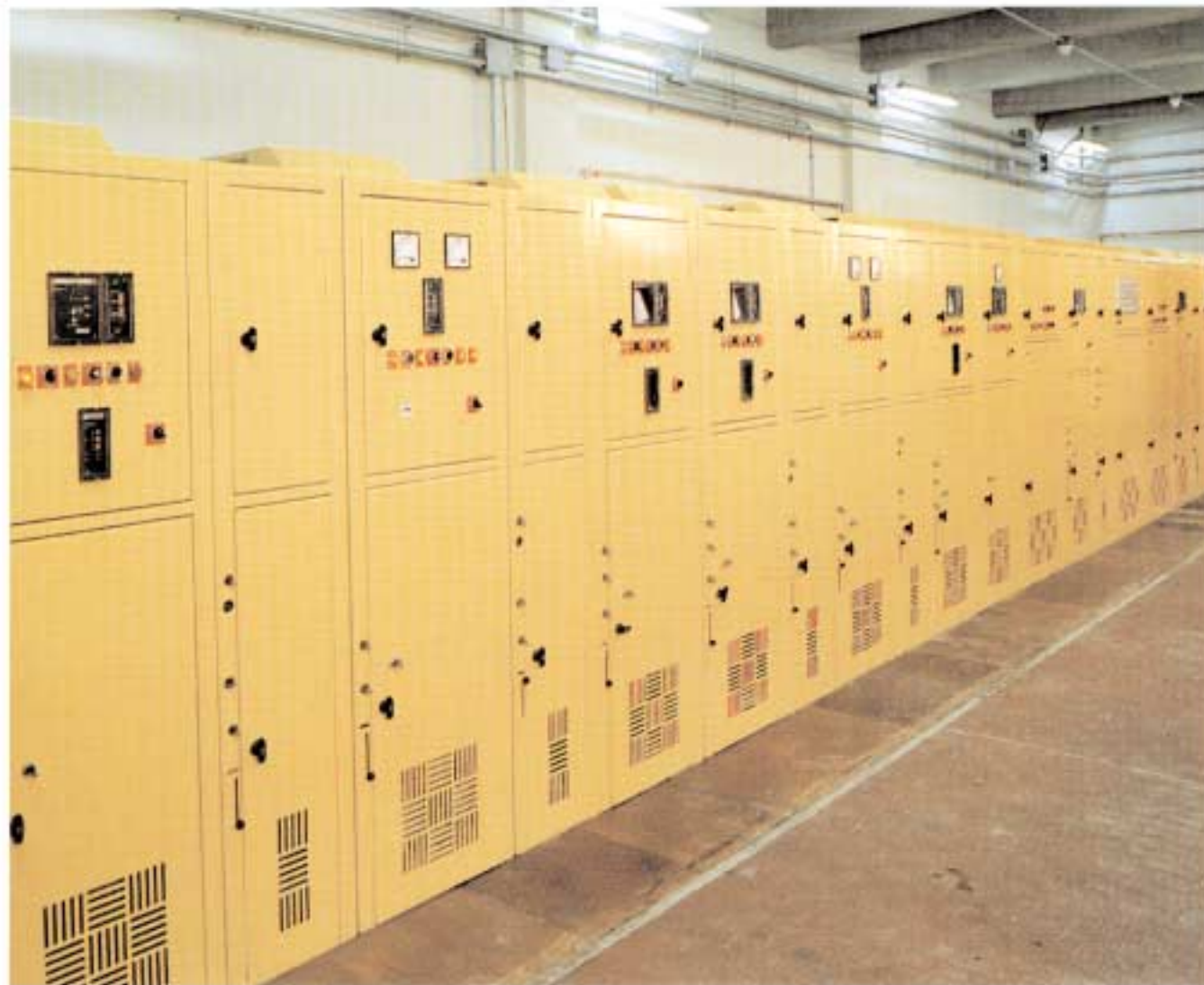
Complete switchgear for subway
